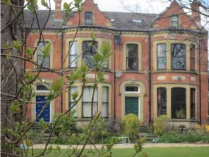
26-28 Spencer Place Leeds, bought in the 1950s by the Leeds Tenants' Housing Society was converted to flats at a time of desperate housing shortage. This venture was the forerunner of Aggrey Housing Society which pioneered accommodation provision for Commonwealth newcomers in Harehills and Chapelton in the 1950s
